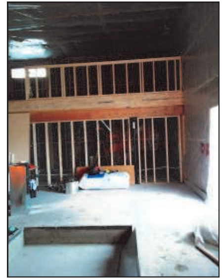
Inside expansion getting framed and ready for drywall. Feb. 2015
